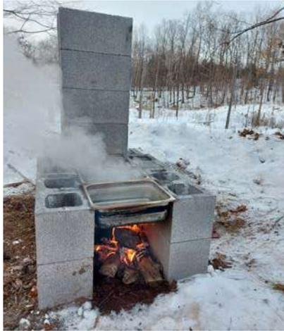
*Our DIY evaporator set-up for 2021. Same three-pan approach: two boiling pans and a warming pan (front) supported by dry stacked (no mortar) concrete blocks.*
