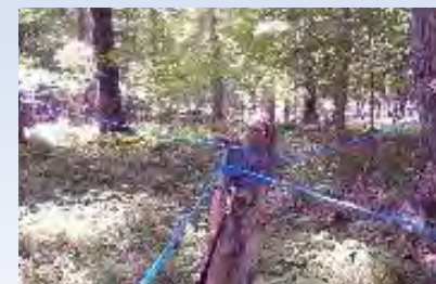
Above: Lateral lines connected to buried mainline in sugar bush
