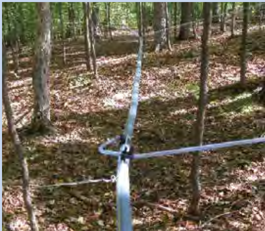
Tubing installation with side wire support
